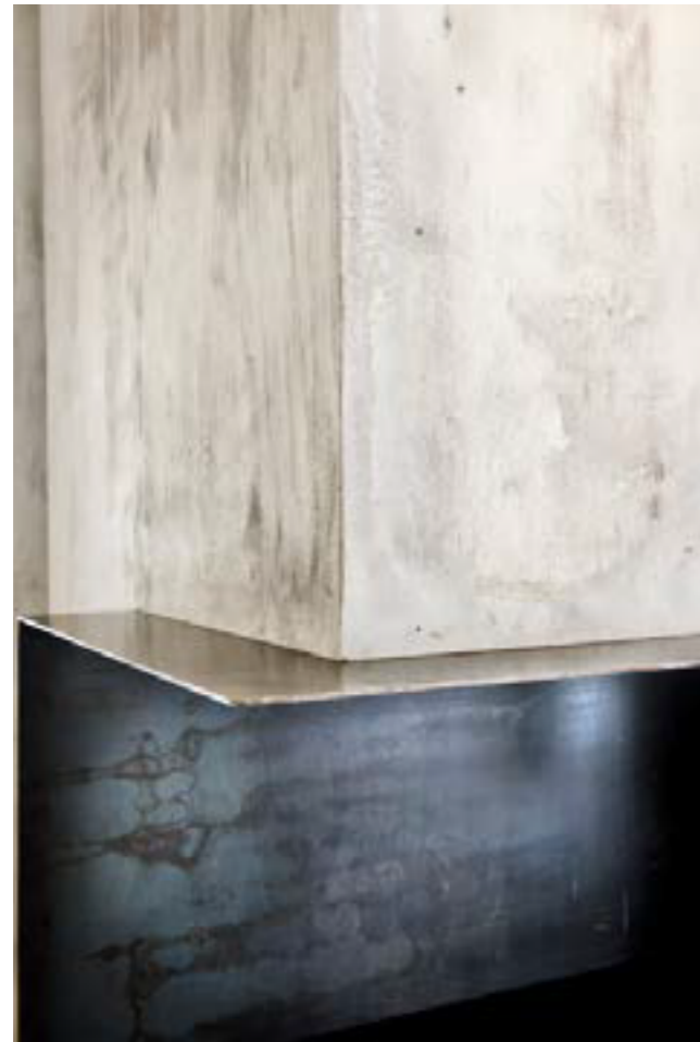
Boiserie rivestita in resina cementizia con nicchie in ferro Cement-resin clad paneling with iron niches
